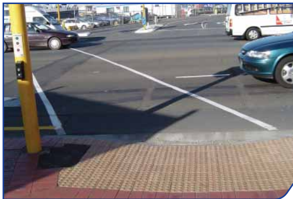
Figure 17 : Visually impaired pedestrians are directed away from the crosswalk by the warning paver layout. Tactile pavers should be laid at the same angle as the crosswalk.
