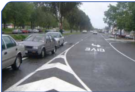
Figure 3 : Captive left turn lane with insufficient warning to motorists.
