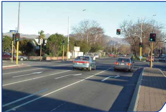
Figure 10 : Fully protected right turn with the required three right turn arrow displays.
