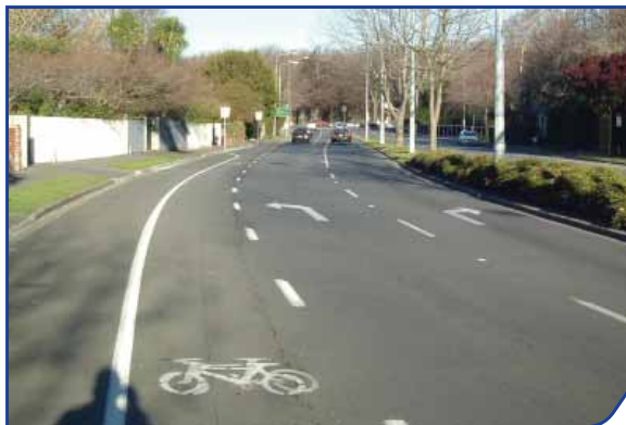
Figure 4 : Lane markings advising motorists of captive turn lanes.
