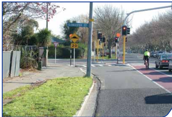
Figure 6 : Slip lane with zebra crossing on raised platform for speed control.
