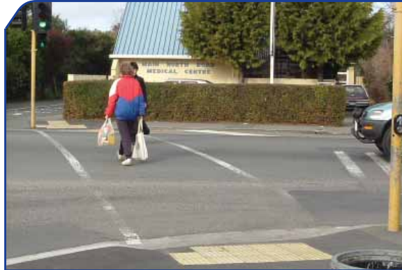
Figure 15 : Bad practice of providing a crosswalk to the right of the side street at a T intersection without pedestrian protection.
