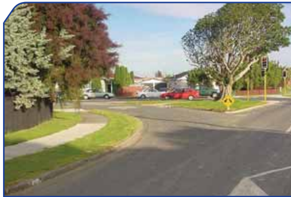
Figure 5 : Pedestrian crossing around the corner – poor visibility.
