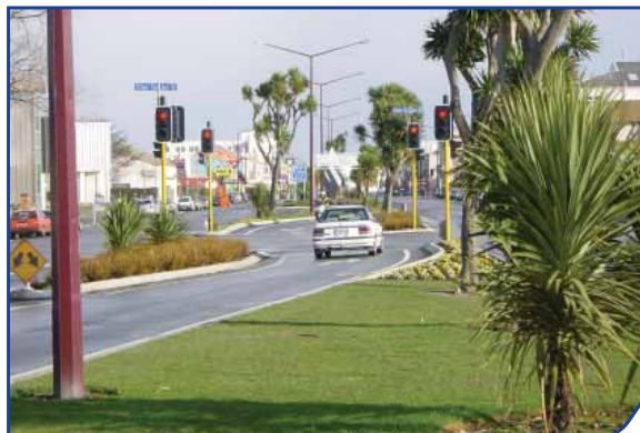
Figure 2 : Right turn bays incorporated into solid median achieving excellent forward-visibility.
