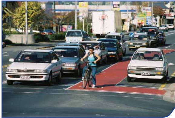
Figure 20 : A good example of providing for cyclists at traffic signals.
