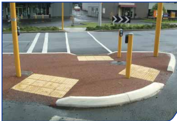
Figure 18 : Use of stub post for appropriate placement of pedestrian call box adjacent to the pram crossing 1 .
