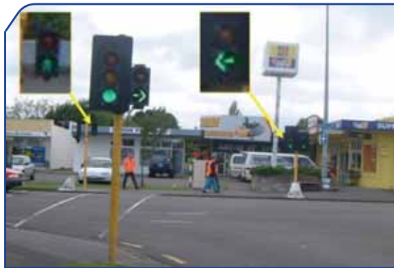
Figure 13 : Non-complying green left turn arrow, as Walk is displayed simultaneously.
