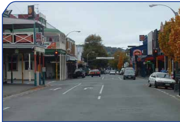
Figure 1 : Offset right turn bays (and hidden primary lantern).
