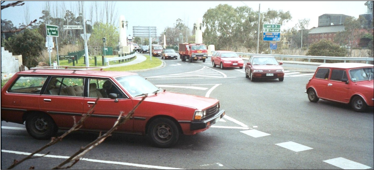
Figure 1 - An example of dominant entry flow at a modern roundabout in Australia (photo modified for driving on the right-hand side of the road)
