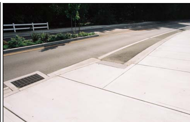
(b) Example of bike entrance ramp Lake Oswego, OR, USA Photo: Lee Rodegerdts
