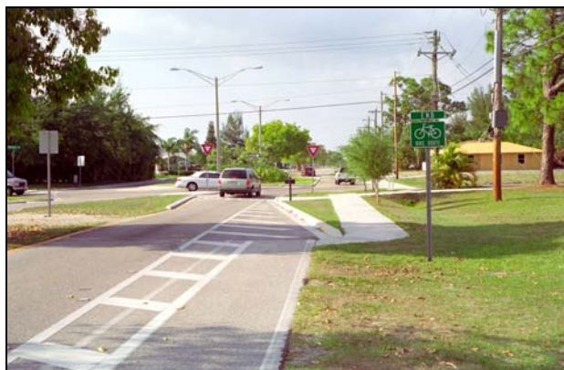
(a) Example of bike exit ramp Cape Coral, FL, USA Photo: Lee Rodegerdts
