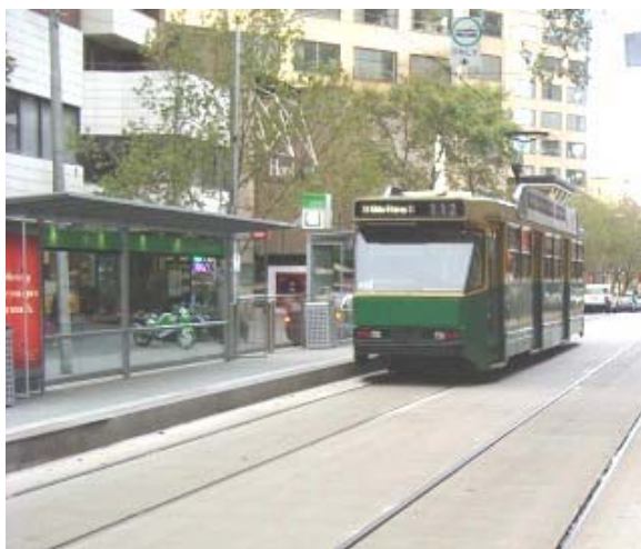
Figure 1: Superstop showing raised platform and passenger infrastructure
