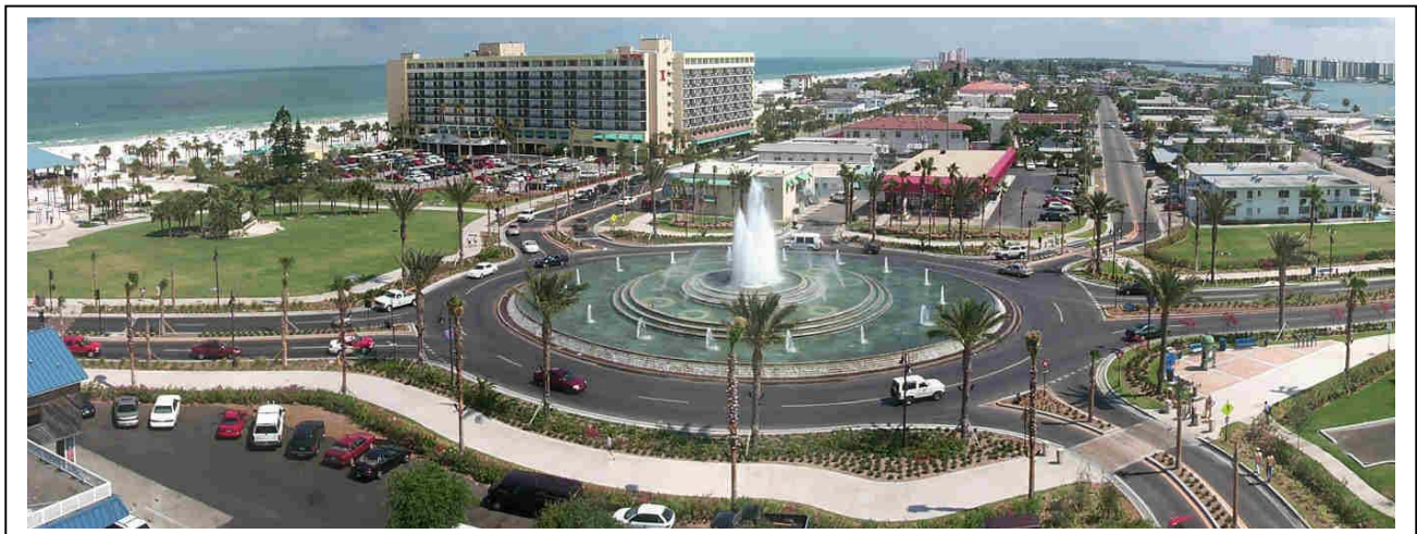
The Clearwater Beach Entryway Roundabout Project. View looking north northwest. Photo by Ken Sides
