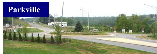
MoDOT’s first two “modern” roundabouts.
