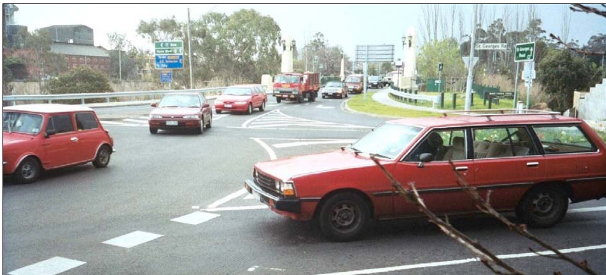
Figure 4.5 - An example of dominant entry flow at a roundabout (Melbourne, Australia)
