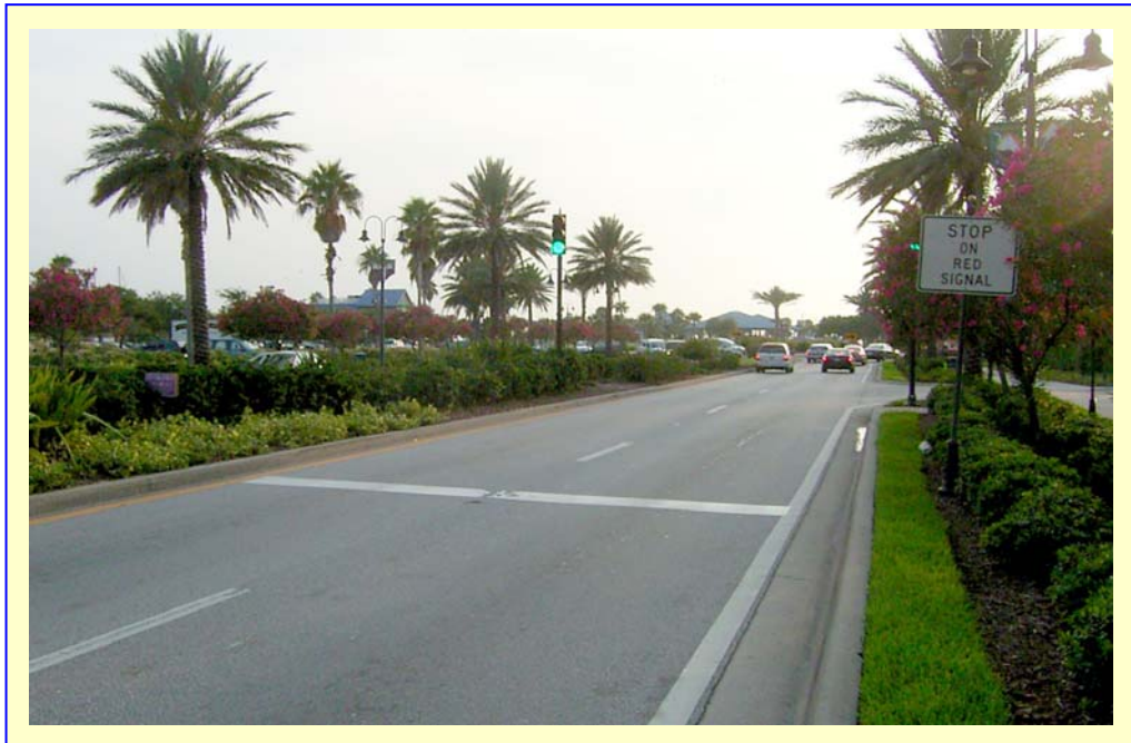
Figure 6 - Metering signals at the Clearwater roundabout, Florida, USA (24)
